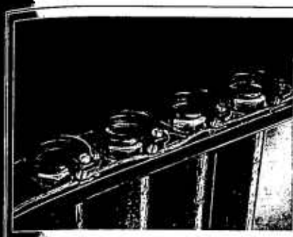
Exhibit 250.35 Grounding bushings used to connect a copper bonding or grounding wire to conduits. (Courtesy of Thomas & Betts Corp.)
