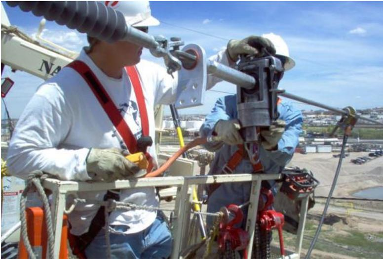
Figure 76 - Conventional 60 ton compression press / die used to complete dead-end (or splice) assembly for ACCC® conductor
