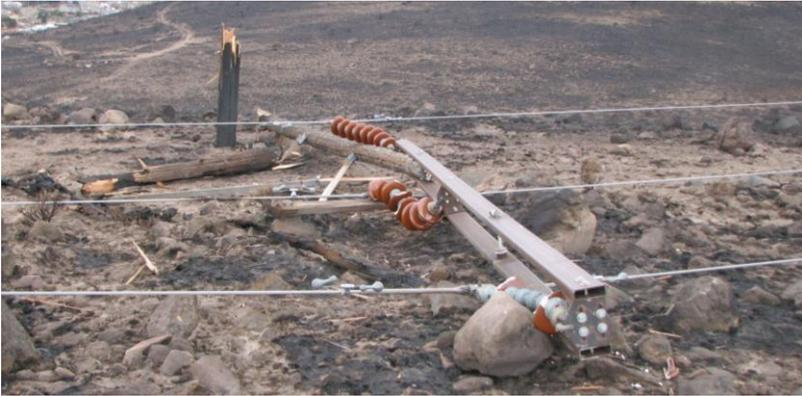
Figure 73 – ACSS<sup>®</sup> Linnet conductor fallen to the ground after 4 wood H-frame structures burned in firestorm near Reno, Nevada. The conductor was undamaged. The H-frame structures and insulators were replaced, the conductors and metal cross arms were lifted back in place and the line re-energized.
