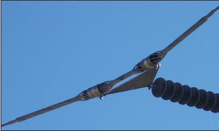
Figure 37 - Double AGS suspension clamp and armor rod.
