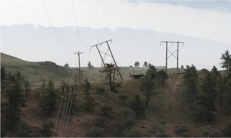
Figure 74 – ACCC Linnet size conductor undamaged due to wind / pole deflection
