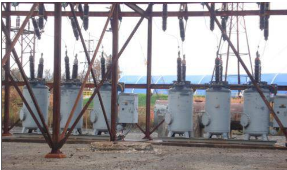
Figure II - Rome Station Structures and Foundations are Severely Deteriorated
