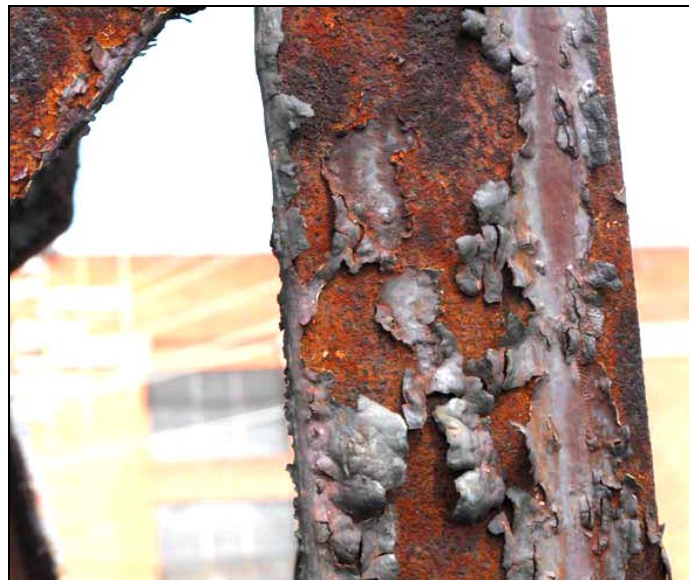
Steel Structures at Lockport are Deteriorated
