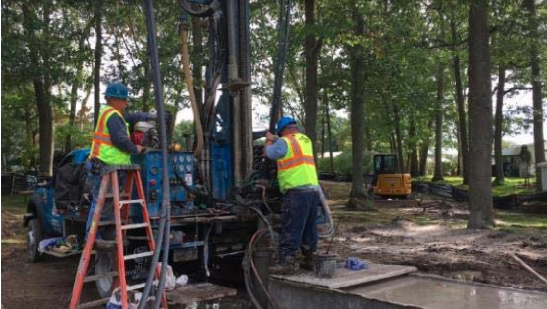
Photo of the geothermal pipes being installed after well boring completion at the Glenwood Village Site.
