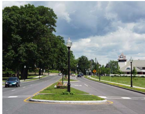
An example of a landscaped median functioning as a gateway and a traffic calming method
