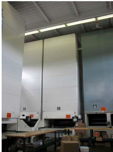
Figure 27: BCW Storage Towers 1001
