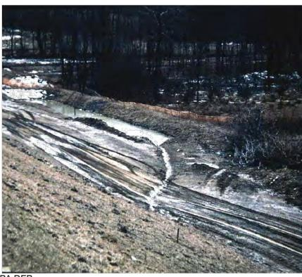
Discharges should be to the downslope side of access roads with a maximum gradient of 3% in the dip. For access roads with grades up to 5%, Standard Construction Detail # 3-6 should be used. Roadways with steeper grades should use Standard Construction Detail # 3-7.
