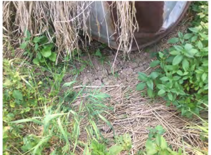
mud cracks near culvert, change in vegetation.
