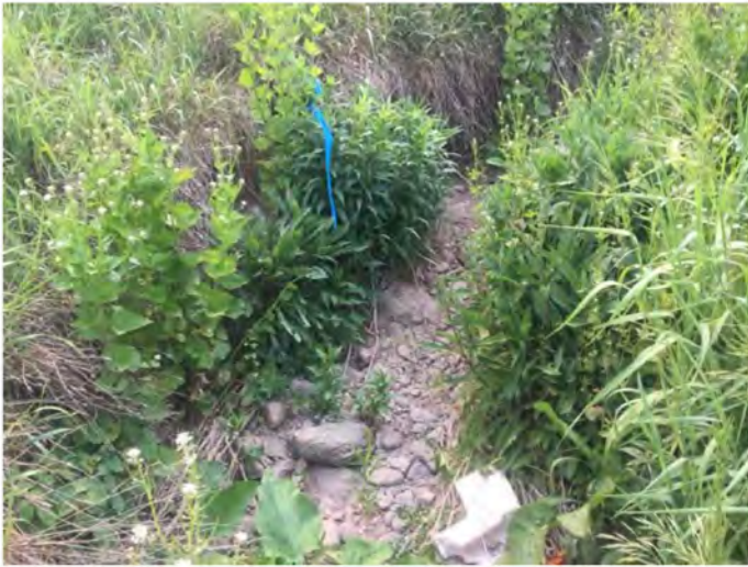
change in vegetation, mud cracks, break in slope
