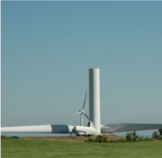
Figure 5.2-6. Turbine Laydown and Assembly
