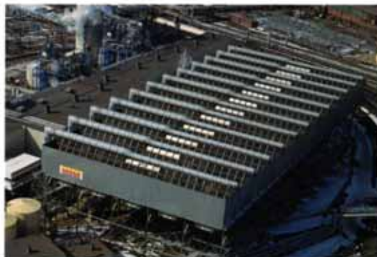
Maui Electric's Maalaea Combined Cycle Plant utilizes the vertical condenser configuration. (left)
