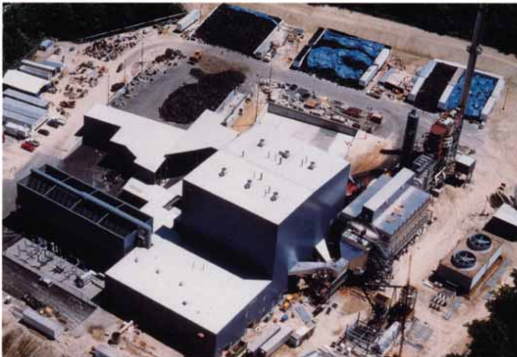
GEA installed a water saving parallel condensing system at the Exeter Energy Resource Recovery Facility in Sterling, Connecticut.
