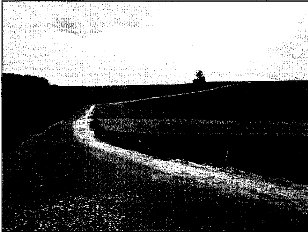
Improved access road to T1A and T2A
