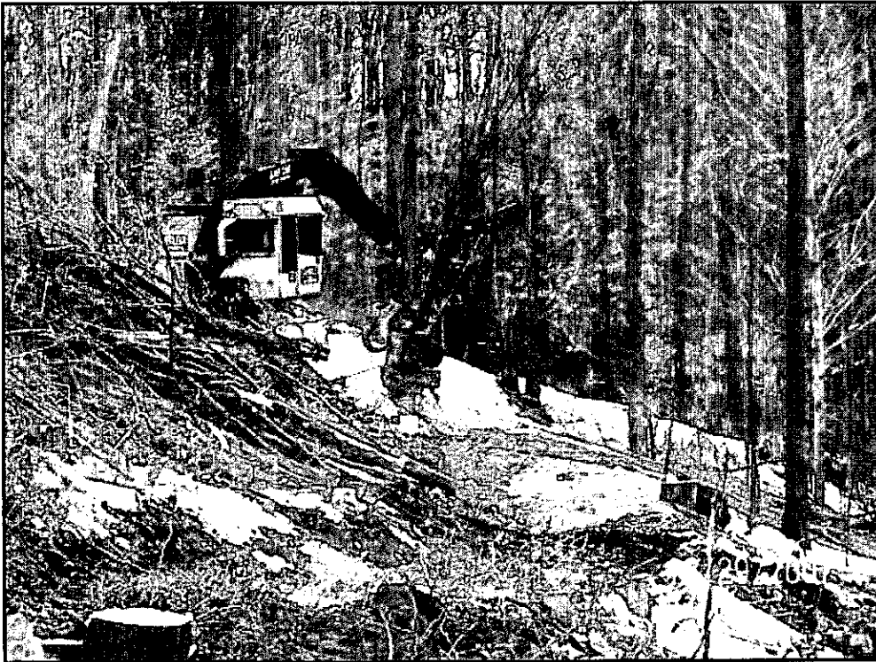
Tree clearing on the 115 kV Transmission Line near State Route 415
