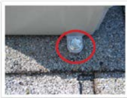
Photo 7: Where not protected from physical damage, equipment grounding conductor must be #6 or larger: NEC 690.46, 250.120(C). Conductors laying on asphalt shingles will become damaged and will not last a PV system's expected 30-year lifespan.
