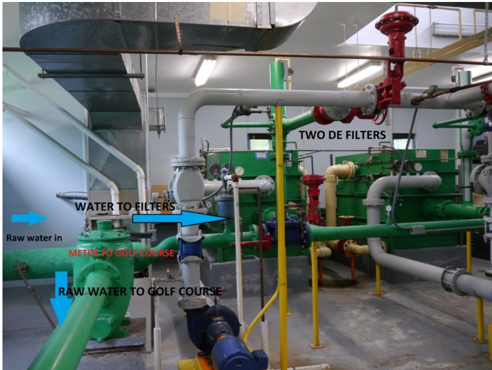
Water treatment plant (above) and finished water pumps (below)
