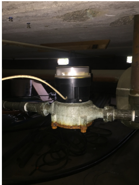
Master meter to the Cottages (above) and sewer treatment plant meter (below)
