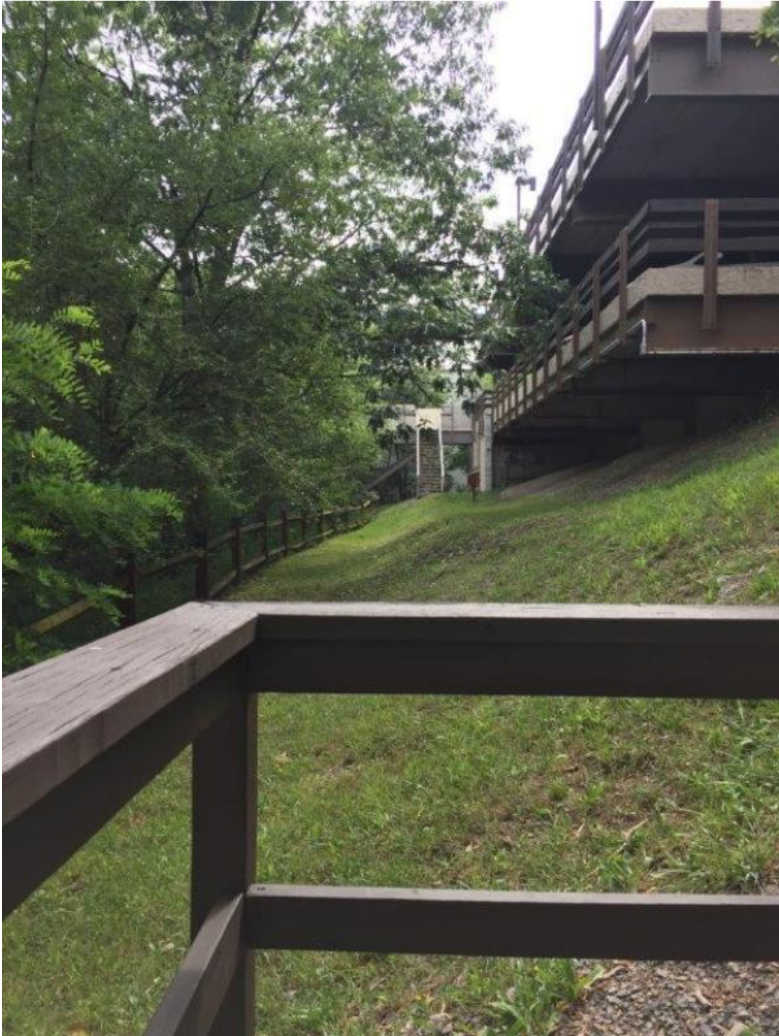
Condo 1 service location (buried underground)
