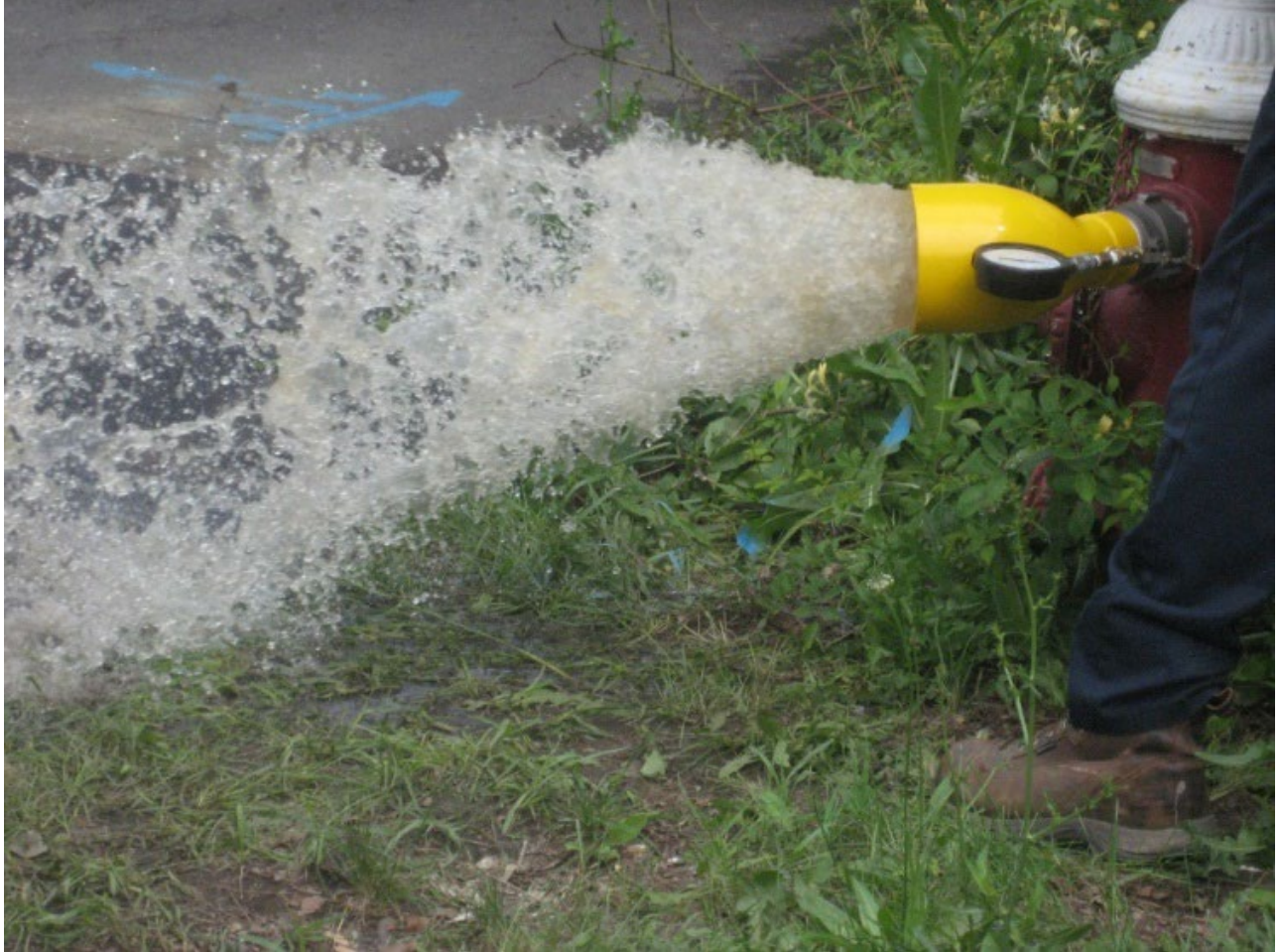
Hydrant 1-89 Flow Test conducted on June 10, 2021
