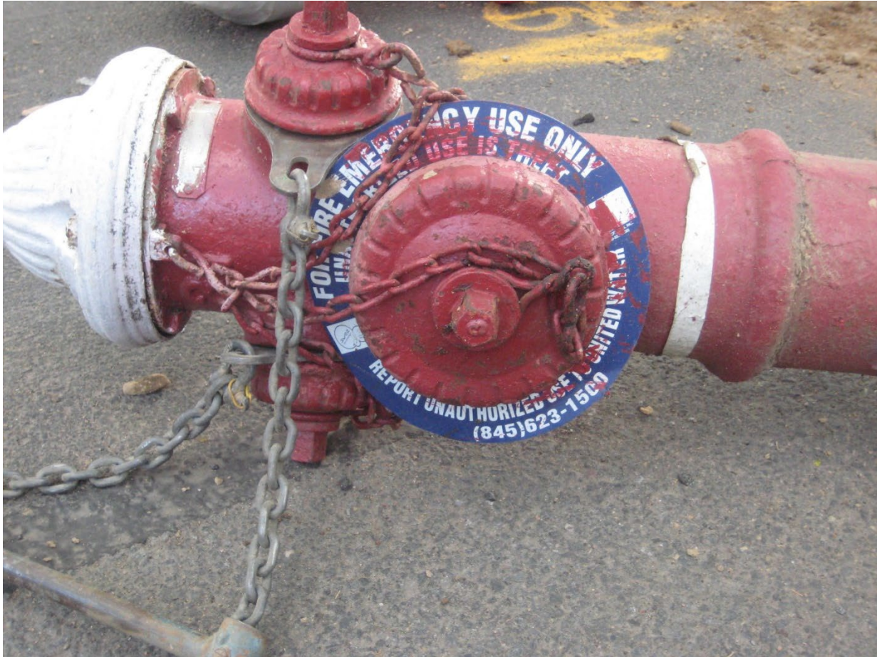
Hydrant 1-119 – Extracted Hydrant Connection Detail Front – April 30, 2021
