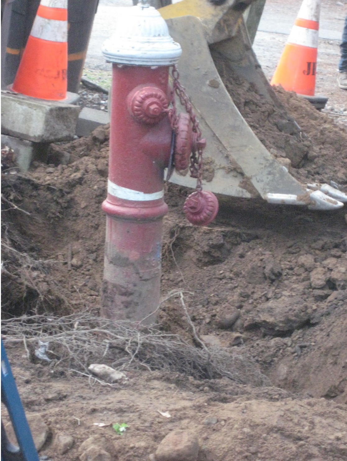
Hydrant 1-119 – Excavated – April 30, 2021
