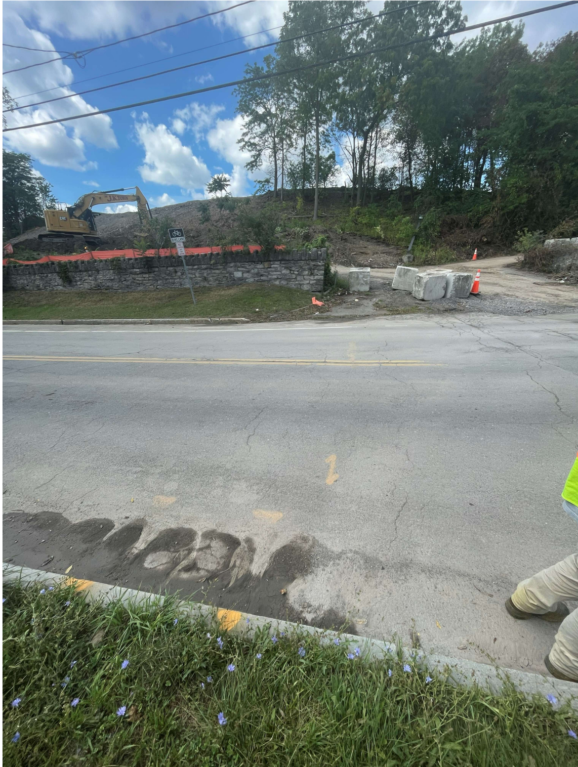
Picture 1: Marks for 4-in plastic main shown on pavement. They turn after the stone blocks and go up to where the excavator is located.
