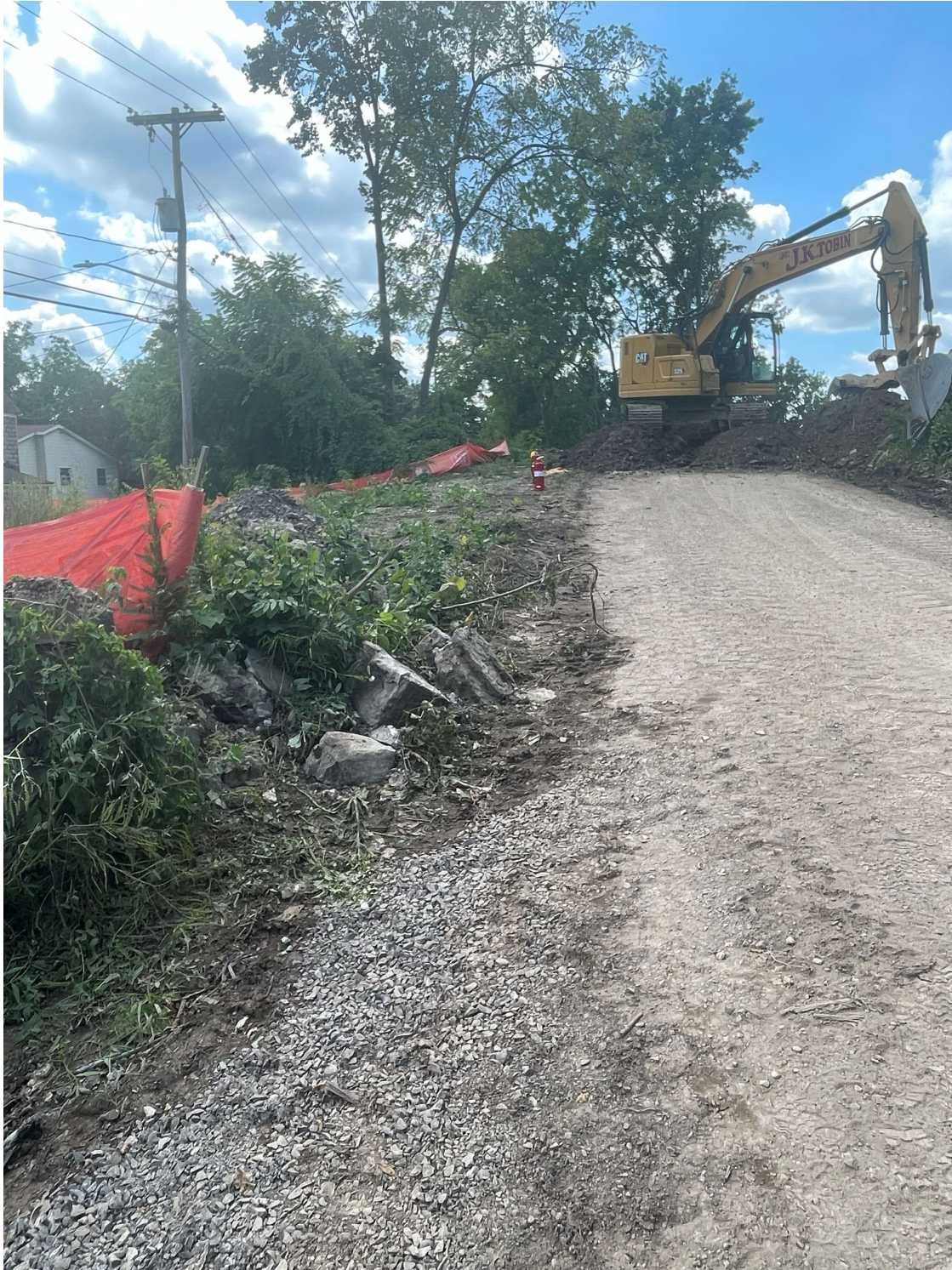
Picture 2: Yellow flags marking the gas main are seen up the side of the dirt road.
