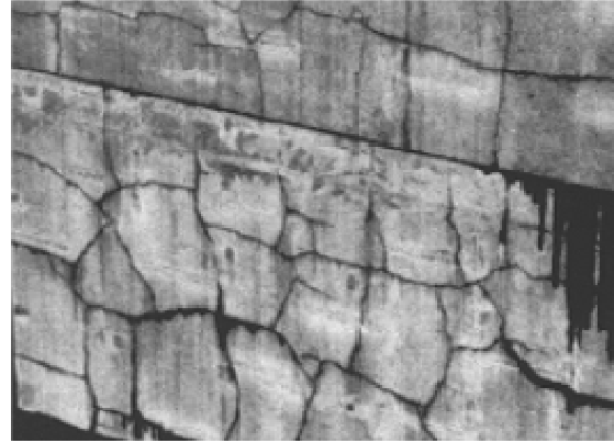
Pattern Cracking
