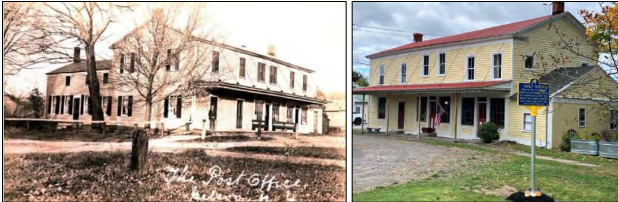
Figure 4. Historic (left) and current (right) views of Old Drover's Tavern (Photographs courtesy of Nelson Preservation Associates).
