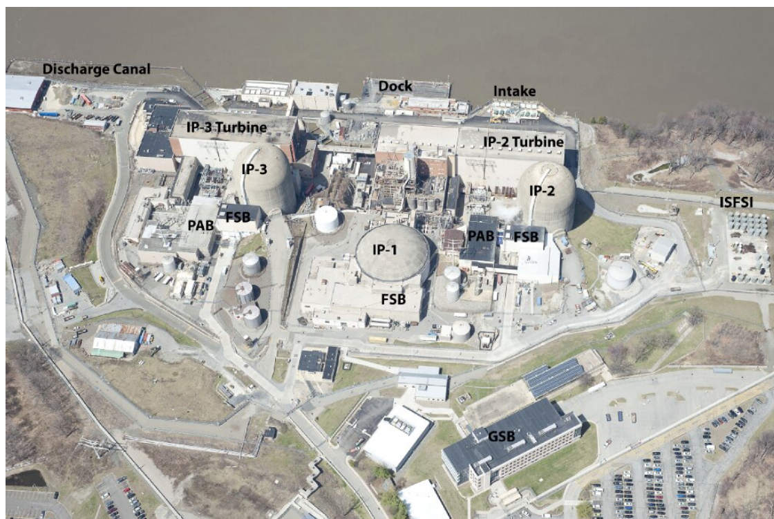
Photo 3: Indian Point Buildings and Structures
