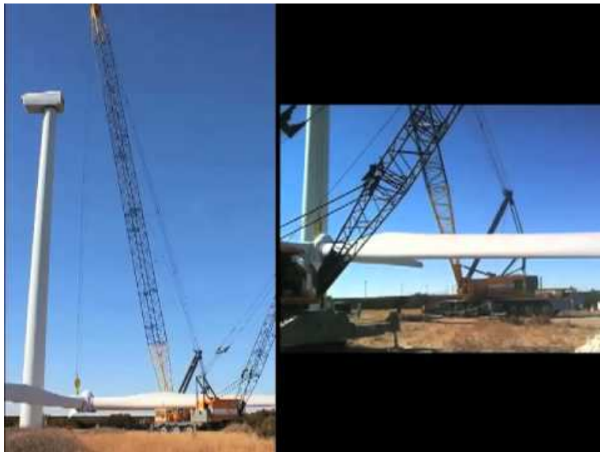
Photo 15: Turbine Rotor Lift
