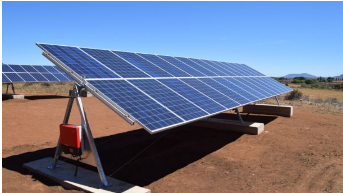
Photo 17: Solar Panel Single-Axis Installation (Photo Credit: Deger energie-Bmbh & Co. website)
