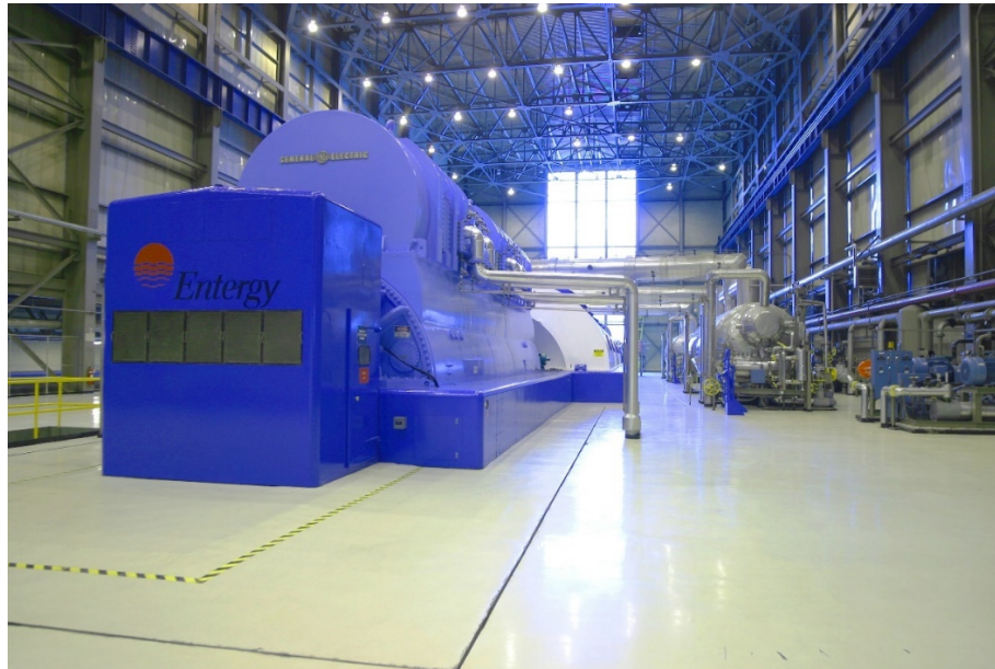
Photo 4: Indian Point Unit 2 Turbine Building
