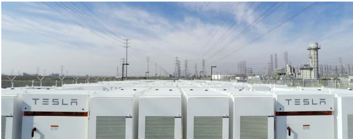
Photo 19: 20 MW/80 MWh Battery Storage - Southern California Edison (Photo Credit, Tesla website)
