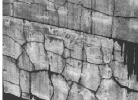
Pattern Cracking
