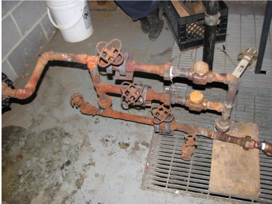
Figure 14 - Photo of Steam Trap Assembly - First Bench Test
