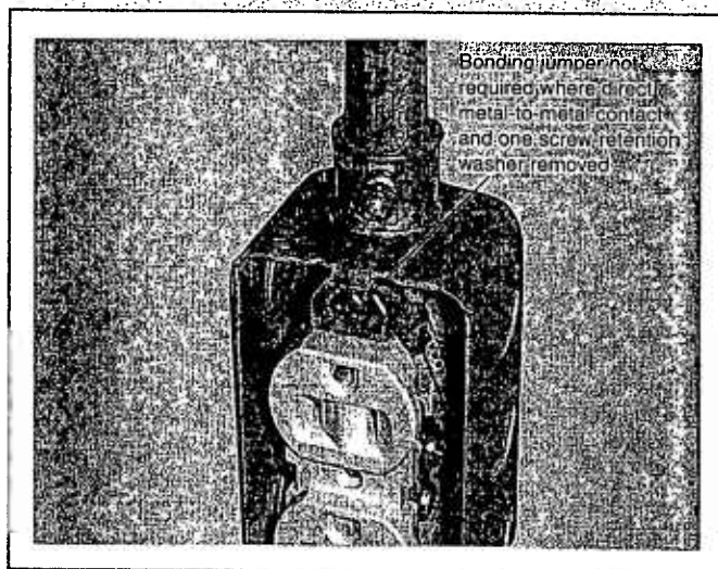
Exhibit 250.52 An example of a box-mounted receptacle attached to a surface box where a bonding jumper is not required provided at least one of the insulating washers is removed.
