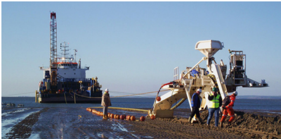
Exhibit 3: Cable ship Stemat Spirit performing a shore-pull using a plough
