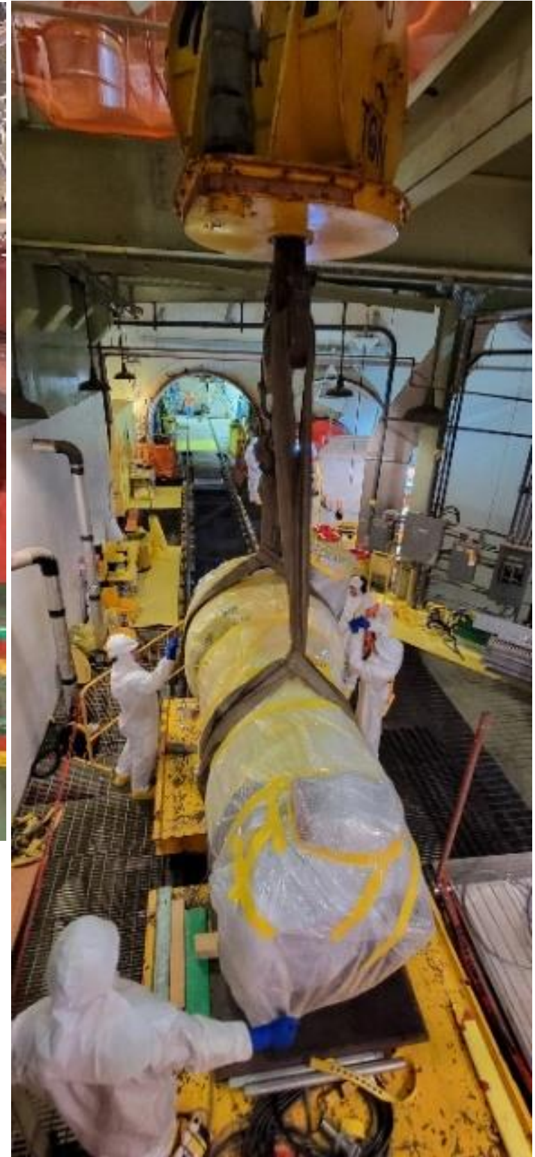
Example of Primary Cooling Pump/Motor packaged out of U1; 4 loop arrangement
