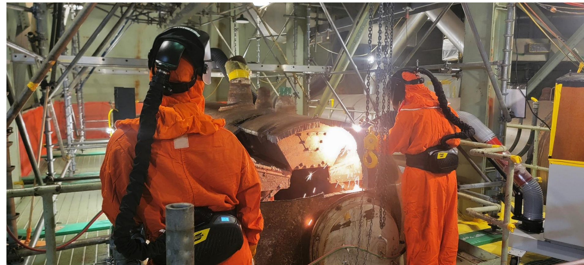
Progress of 11 Boiler Steam Drum Segmentation
