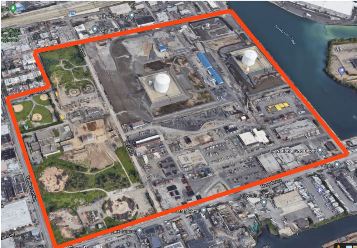
Figure 2-1: Aerial view of the Greenpoint Energy Center
