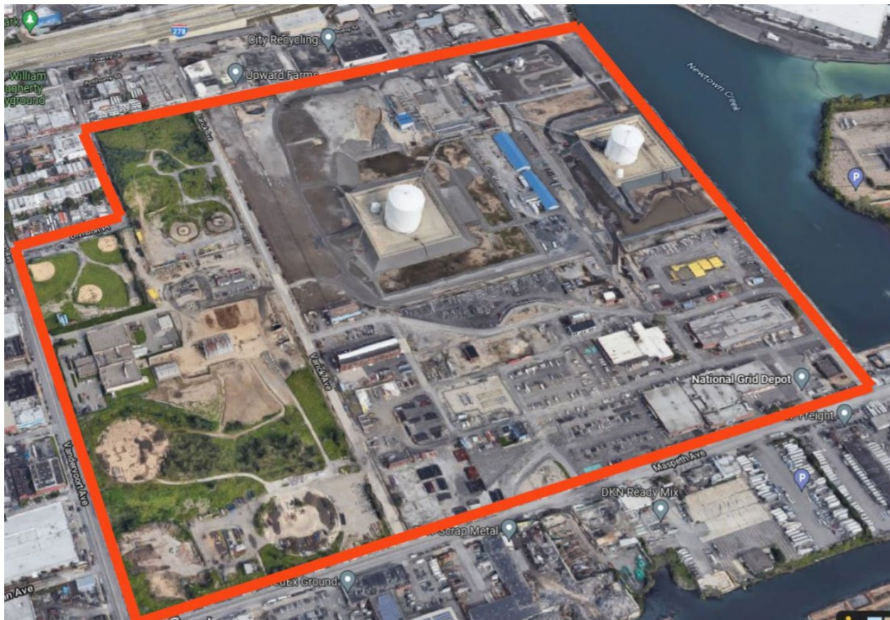
Figure 7-1: Greenpoint Energy Center
