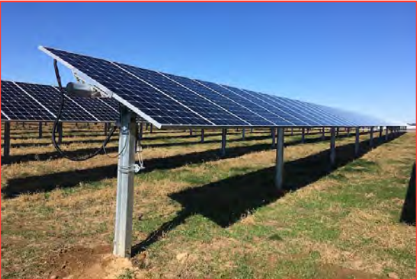
Figure 2: Example of Single-axis Tracking System, Ground-mounted Solar PV
