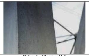
Rating 1 - "Serviceable" Fully painted – overcoat and undercoat intact Fully galvanized – coating intact
