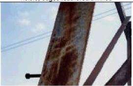
Rating 3 - "Light Corrosion" Very light surface corrosion, majority of coating intact
