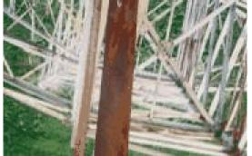
Rating 4 - "Light Pitting" Some very light edge roughening. Loss of greater majority of coating and zinc layers. Corroded surface would dominate surface preparation - remedial action using wire brush, scraper and brushed paint not sufficient to give greatly increase life
