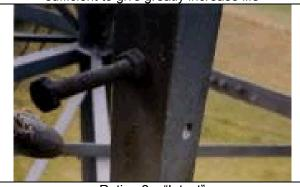
Rating 2 - "Intact" Paint coating over all surface - overcoat may not be intact and some very small areas (<1%) of light corrosion may be present. Galvanizing intact except for some very small areas (<1%) of light corrosion
