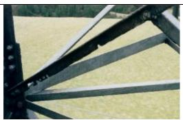
Rating 6 - "Very Severe Deterioration" Perforated Element – severe physical damage
