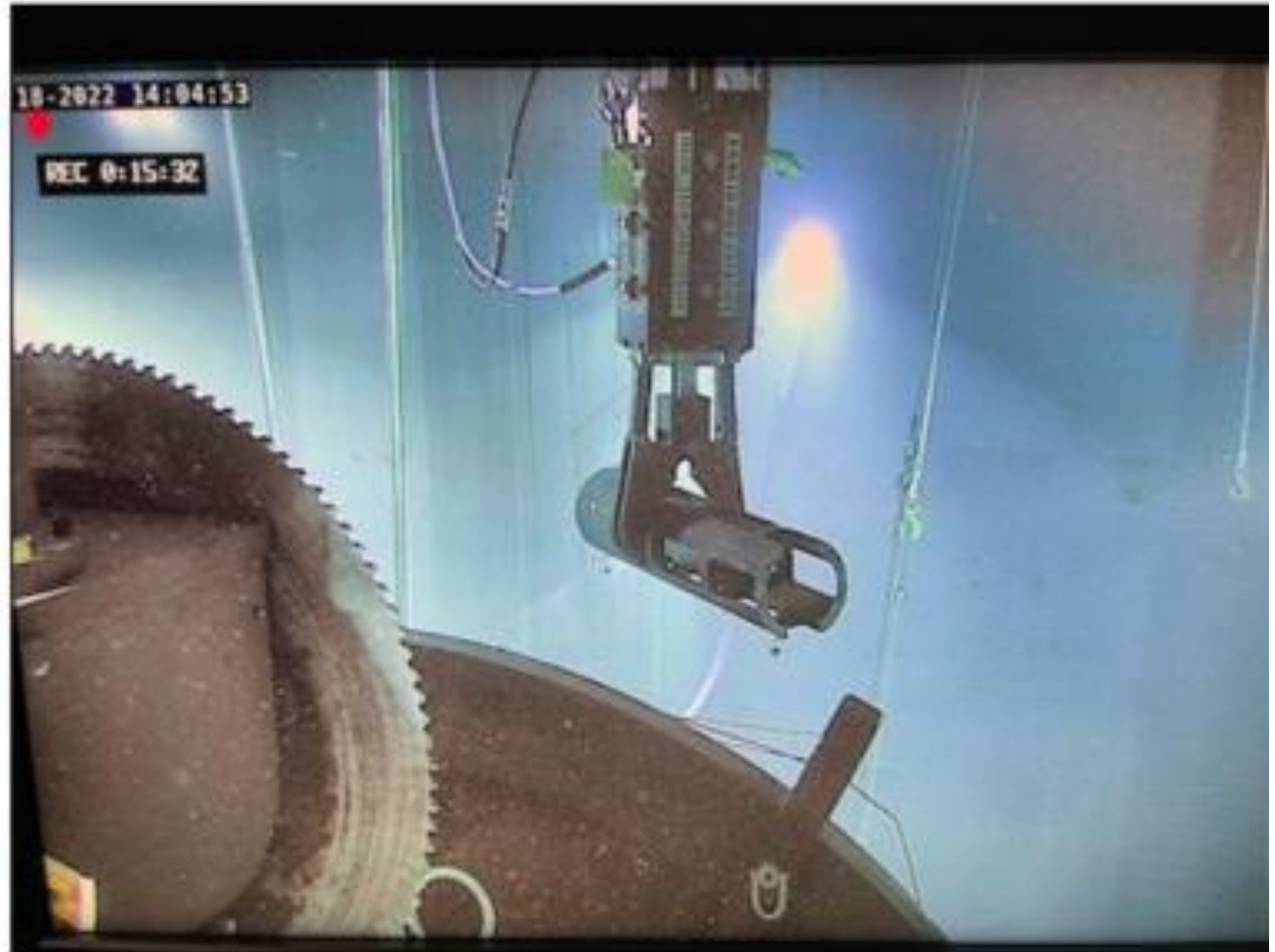
Section of CRDM column segmented from Upper Reactor Vessel Internals
