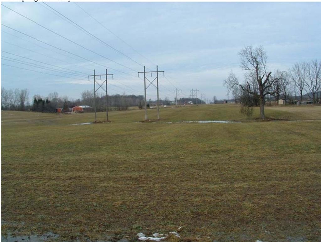
Figure 4-6 Existing NYSEG ROW looking north at Reyer Road
