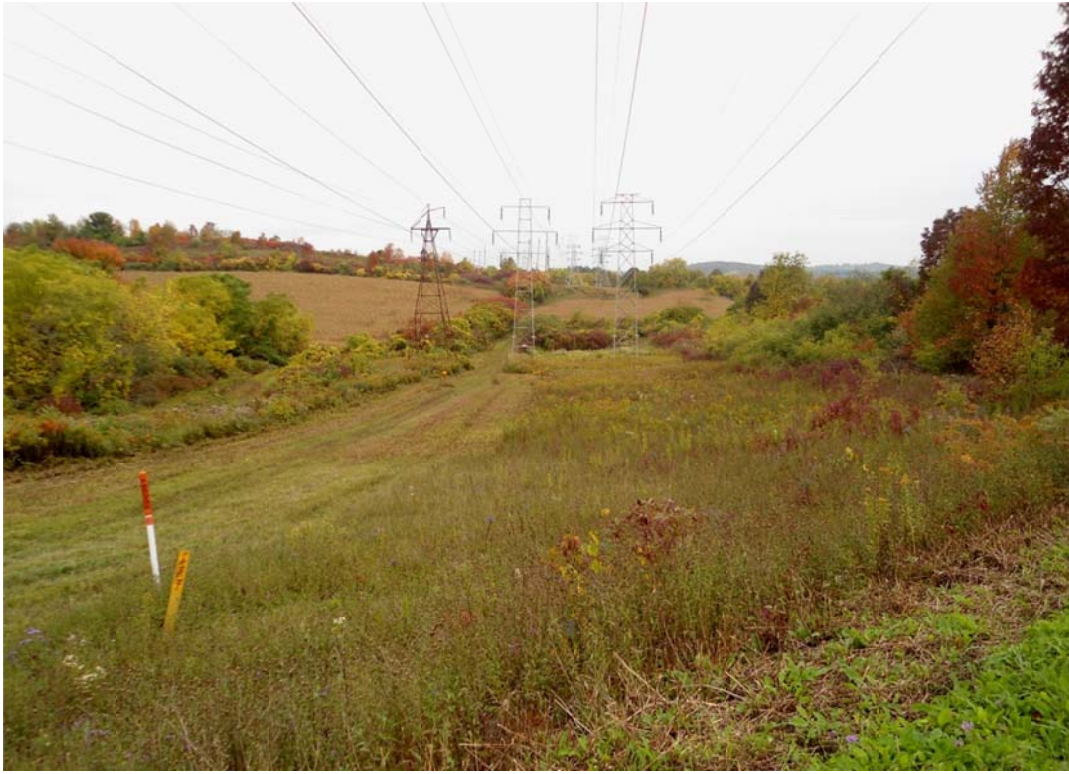
Figure 4-14 Existing National Grid ROW looking west near Kingston Road
