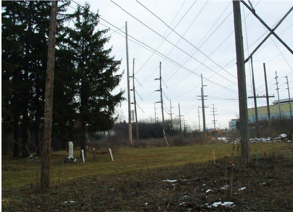
Figure 4-4 Existing NYSEG ROW looking northwest from State Street Substation toward the Cold Springs Cemetery
