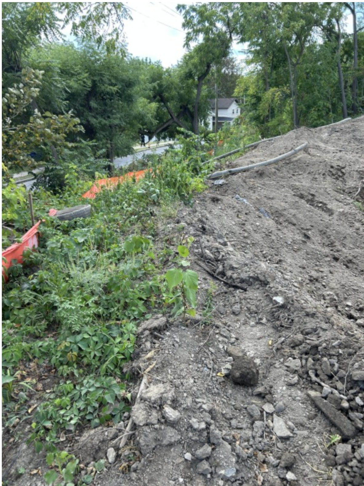
4-inch Plastic service pipe removed uphill of active stub
