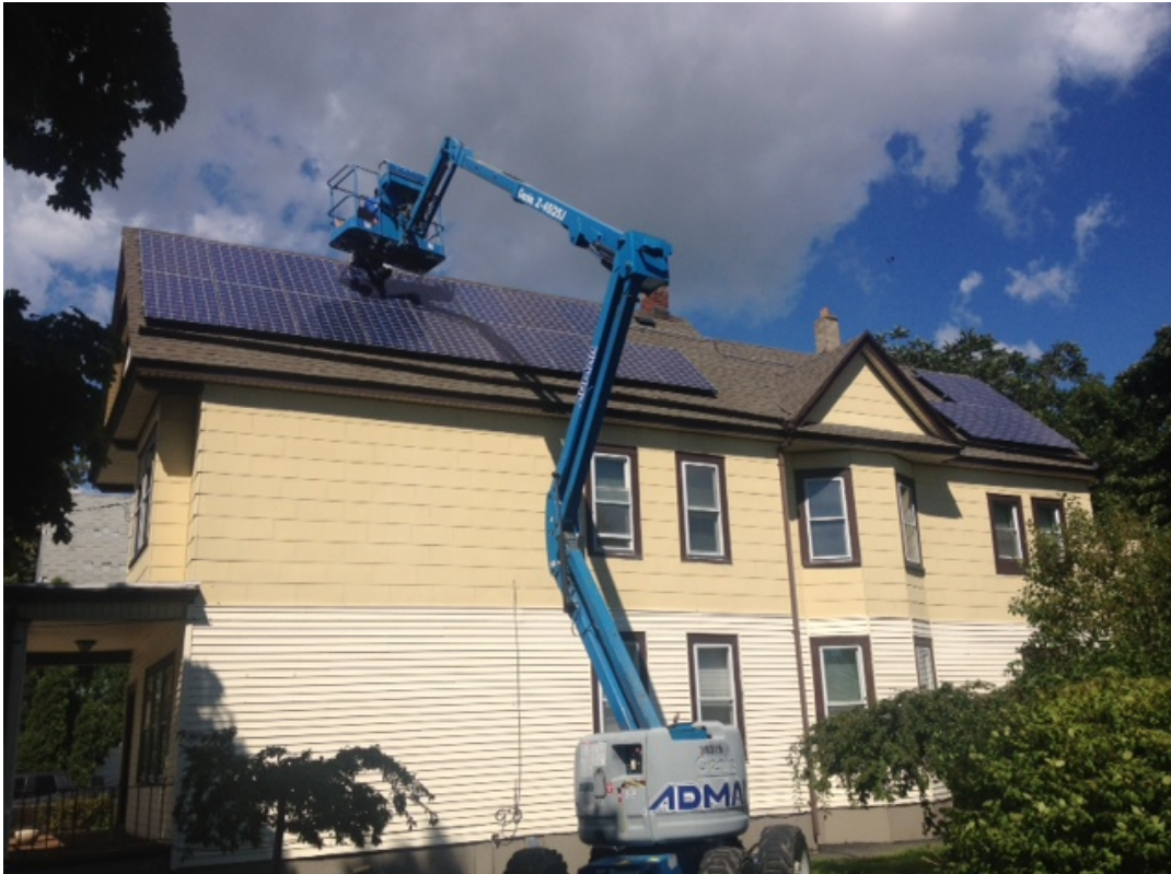
Figure 3-2: Installing the second rooftop solar PV system in the Fruit Belt neighborhood
