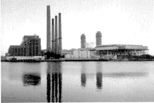
Mystic Station power plant located outside Boston, which was purchased by Constellation Energy this week. (Photo: Business Wire)
