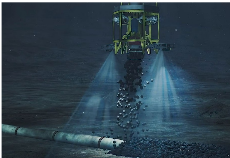
Figure 6-9 Typical subsea rock berm installation with a fall pipe vessel ( www.vanoord.com )
