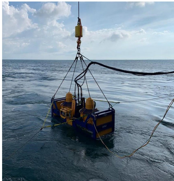
Figure 4: Typical Mass Flow Excavator (MFE)
