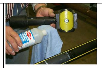
Position tapping tee in center of the scrapped area. Secure the fitting to the pipe in the following manner. NOTE: A separate, reusable installation kit is required. It is unique to the base pipe size. It contains a undersaddle clamp for 2" fittings and a Nylon belt strap for 4", 6" & 8" fittings.
