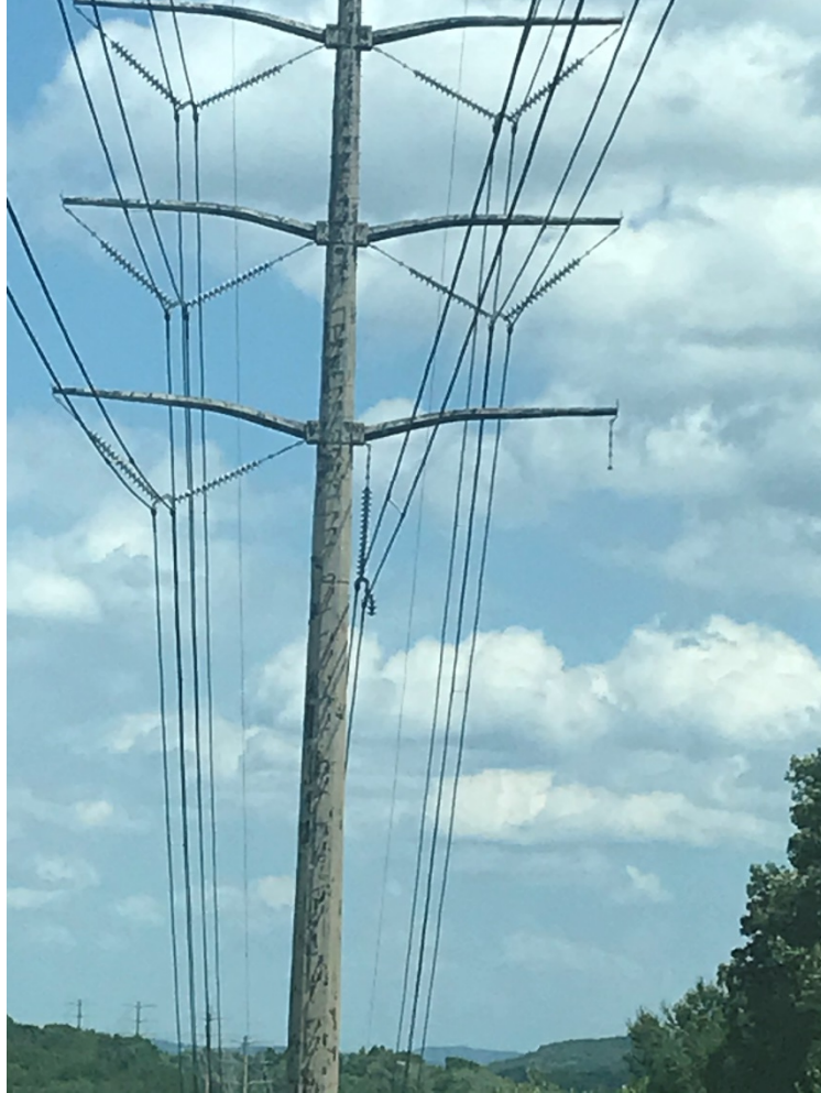
Photo 9 - Transmission tower 345 kV Lines 67/68
