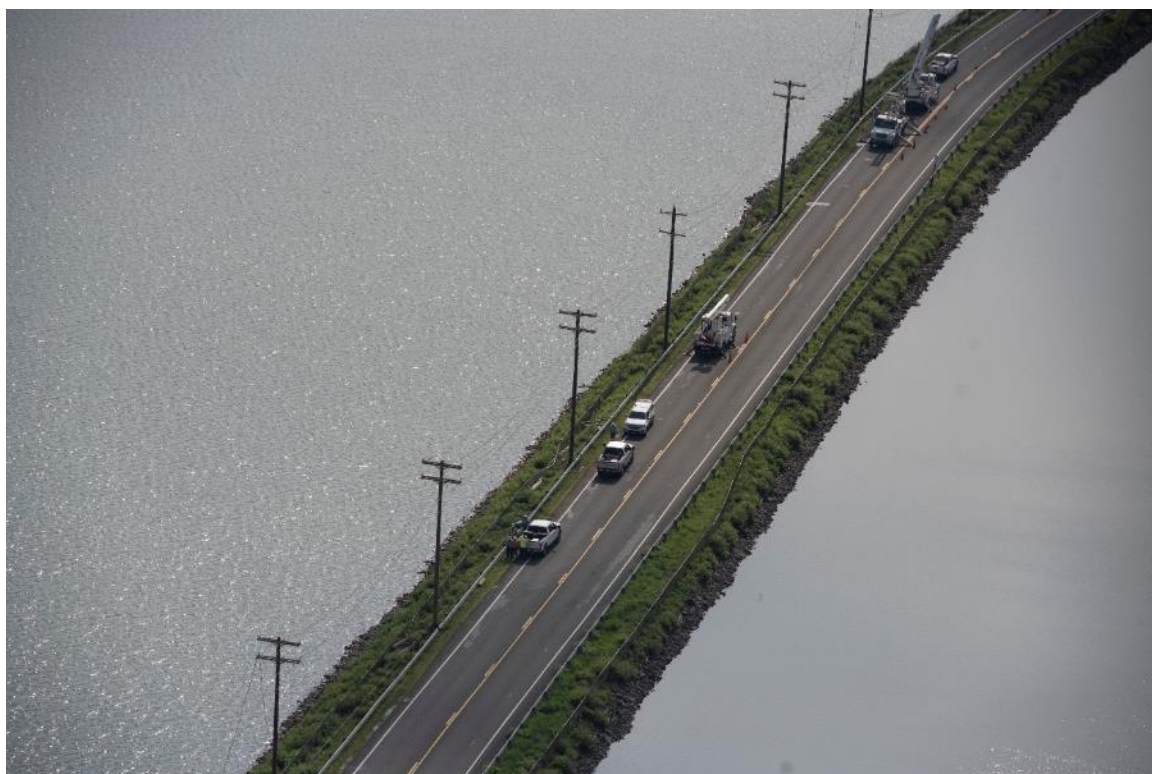
Photo 2 - Contractor repairing double circuit pole line along the causeway over Lake DeForest.
