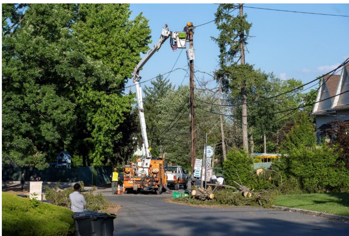
Photo 5 - Damaged transformer, downed trees, Fanley Avenue, Spring Valley
