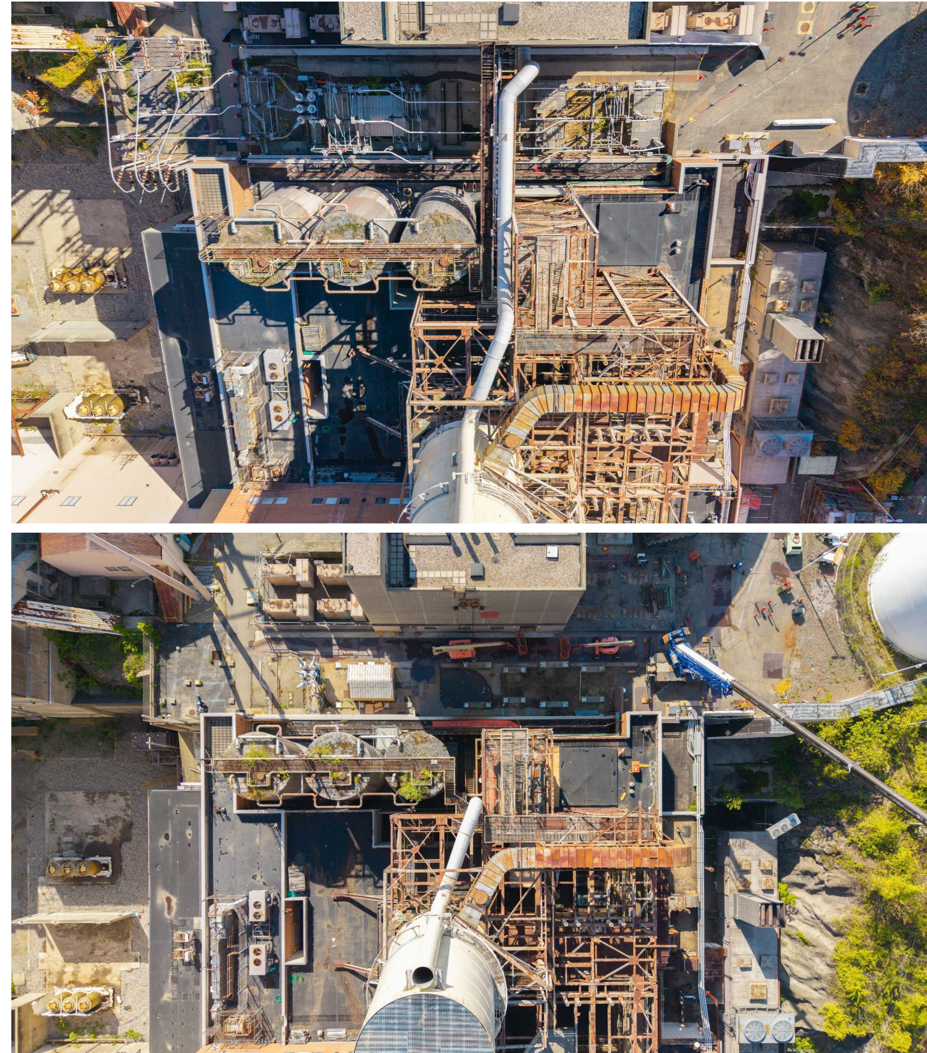
Picture: Aerial view of the Unit 1 Superheater structure
