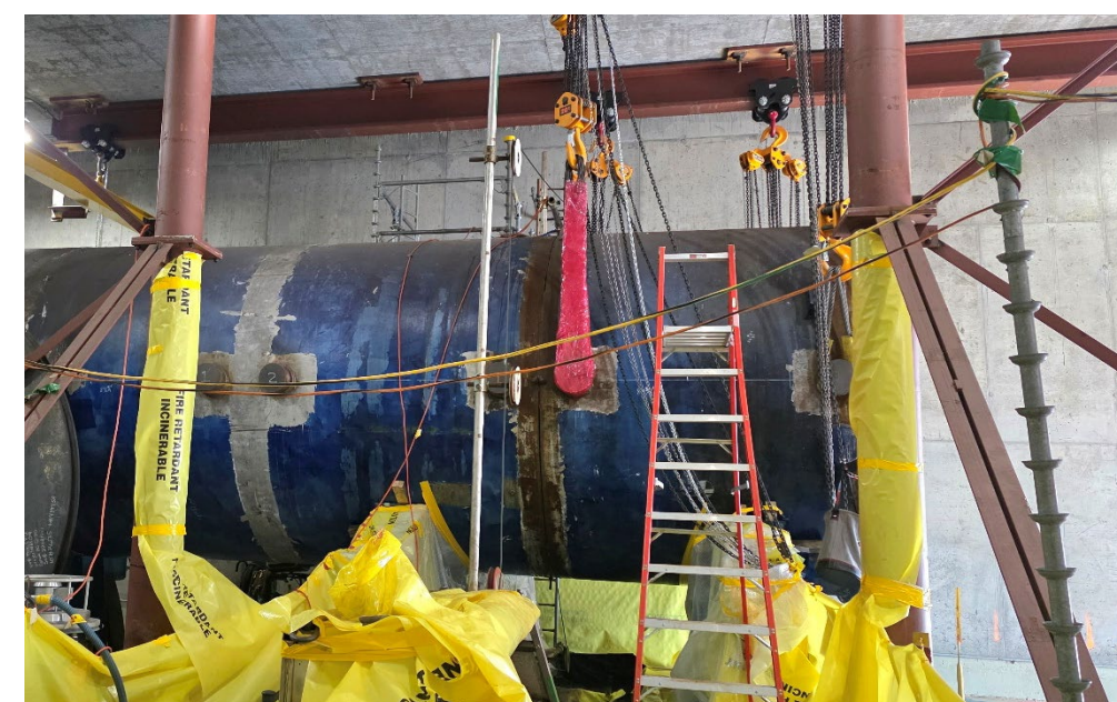
Mausoleum 21 SG Segmentation & Receipt of a SG Section in Texas
