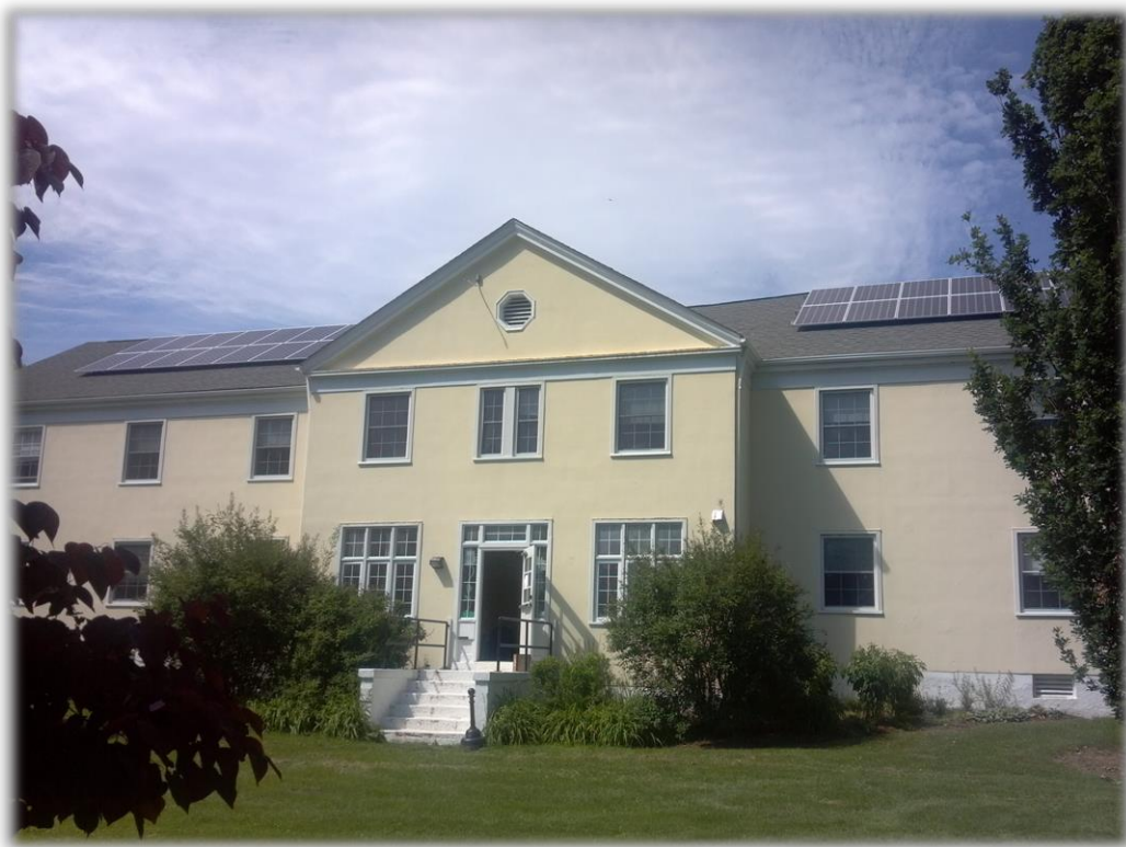
South Hall Dorm with 9kW solar PV array ( Dan Smith, 2014 )
