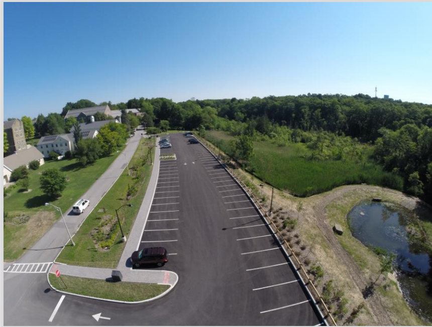
Olin Parking Lot, Bard’s 2015 permeable asphalt parking lot designated for Commuters only, with reconstructed wetland and drainage system. ( LRC Associates, 2015 )
