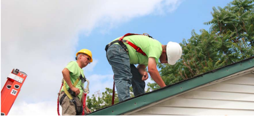
Figure 3-4: Use of safety harnesses by all roof workers is one of several safety protocols followed by the contractor's field installation crews.
