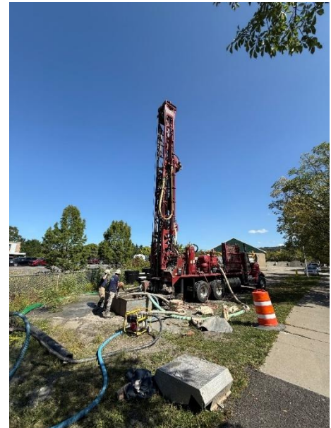
Figure 200: Drilling Production Well #1
