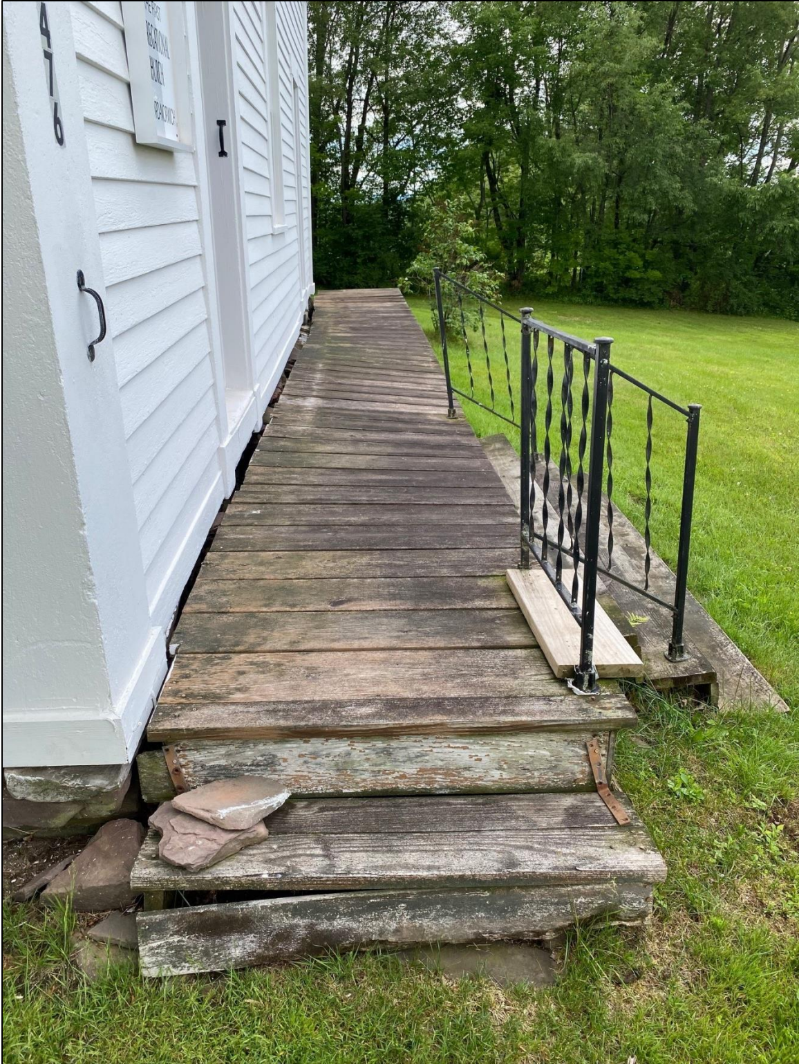
Inset 2.3-7. Deteriorated wood steps and walkway, North Guilford Church.
