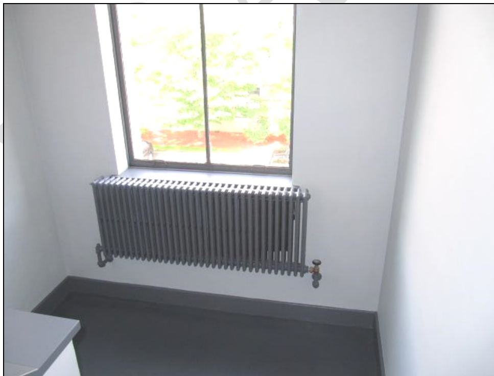
View of Stairway Between Third and Second Floors
