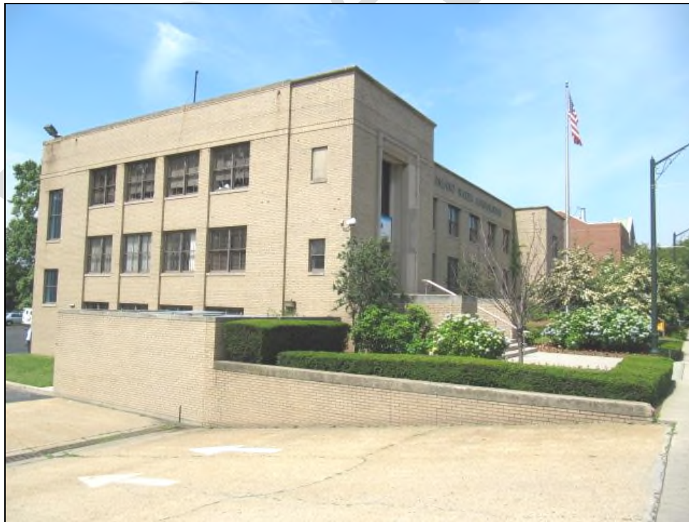
View of East Side of Subject Building and Pump Enclosure from Front Driveway
