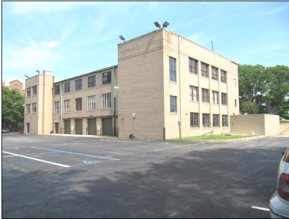
Rear View of Subject Commercial Building Looking Northwesterly from Parking Lot
