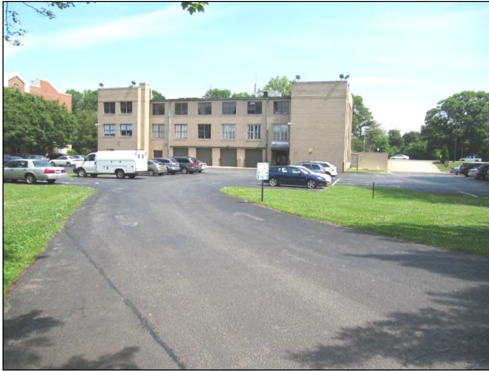
Rear View of Subject Commercial Building Looking Northerly from Rear Driveway
