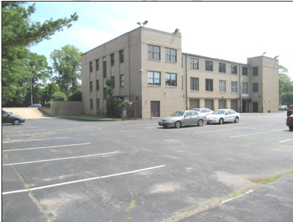
Rear View of Subject Commercial Building Looking Northeasterly from Parking Lot
