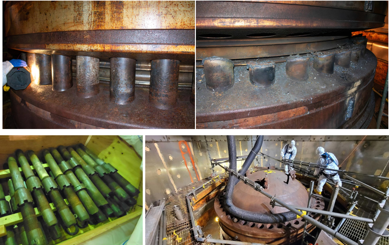
Top: U1 Reactor head bolted and following cutting of the studs Bottom: U1 Reactor head studs and overhead view of head on vessel
