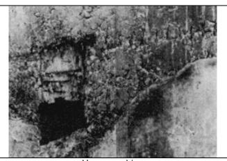
Honeycombing Construction faults, poor workmanship
