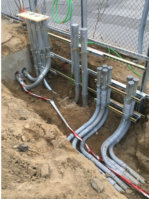
Figure 1: Laying of Charger Electrical Conduit, November 2018
