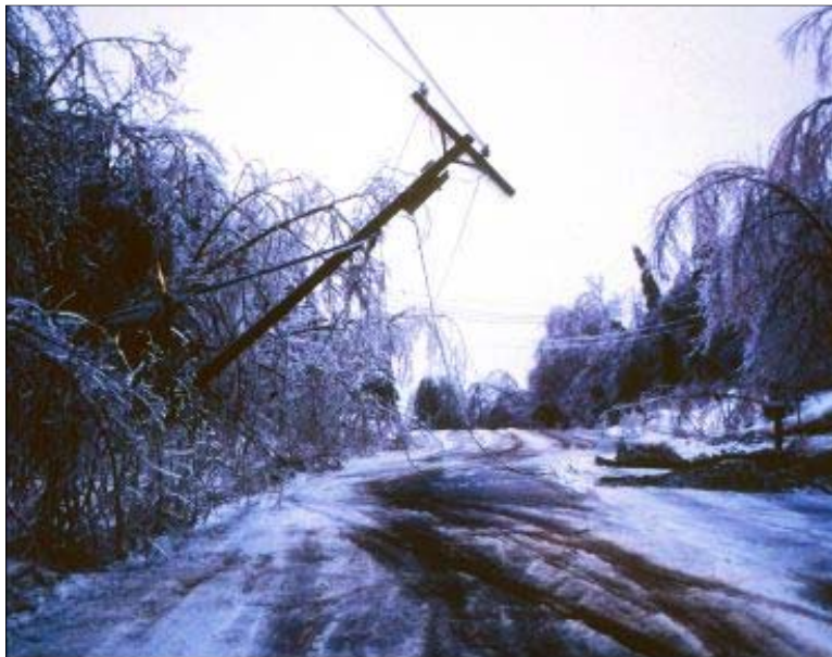
Image 1.1 – Photo of upstate New York after the 1998 Ice Storm 1
