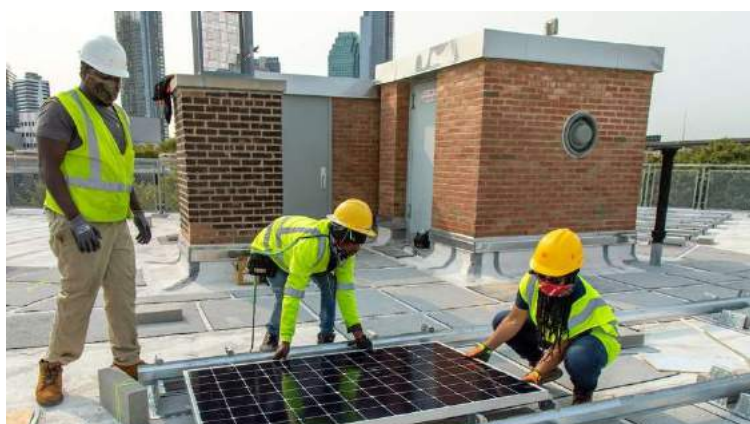
Image 8. Workforce trainees install solar on affordable housing development in Queens, NY. Photo credit: Sunwealth.
