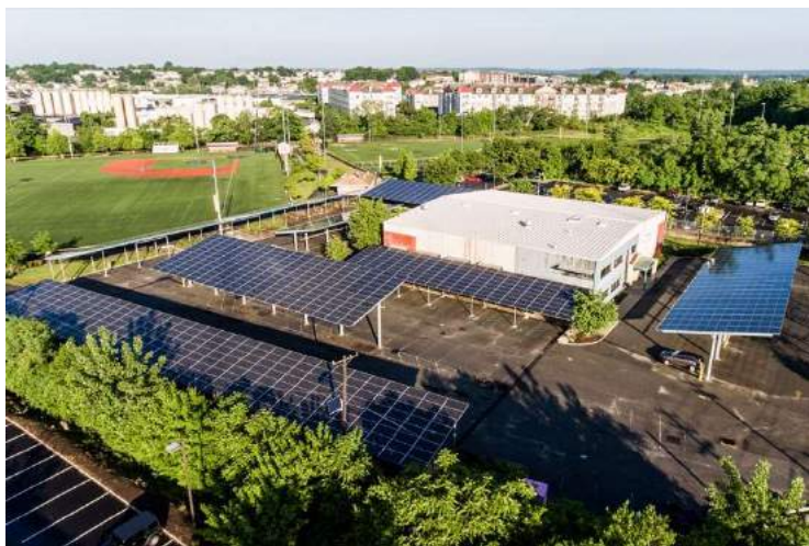
Image 10. Solar carport installation. Photo credit: Ecogy Energy.
