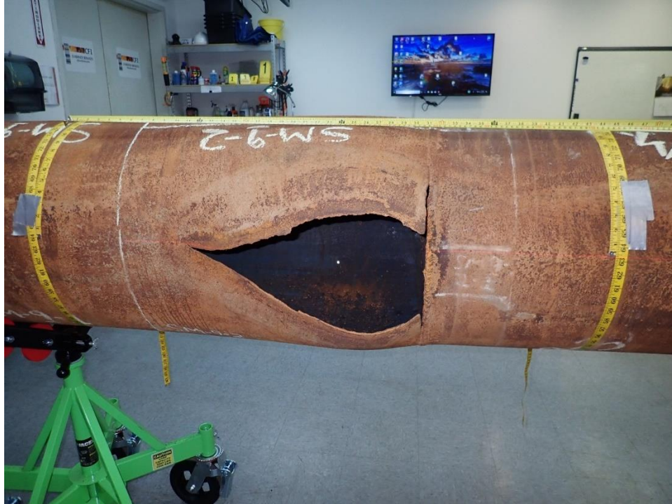
Figure 9 - Close-up of Rupture on Pipe, Taken by Affiliated
