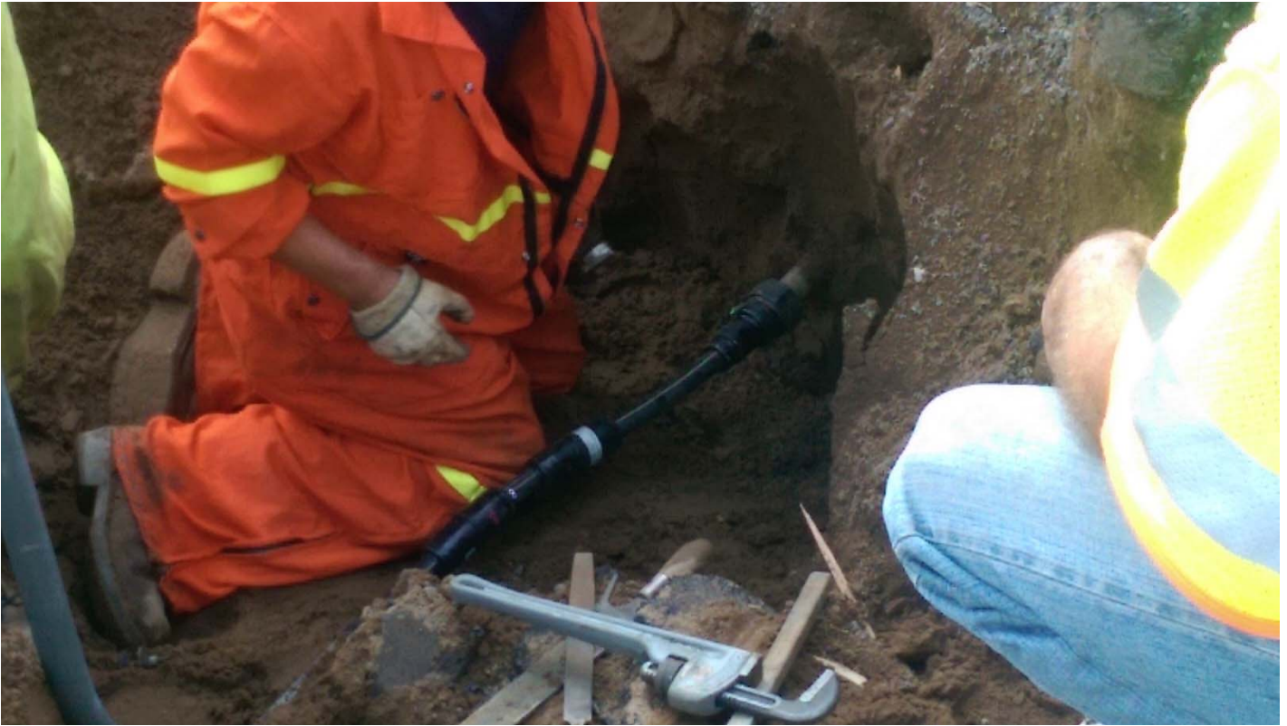
Photo 13 (8/10/14) – National Grid crews pressure testing the service pipe (near the main).
