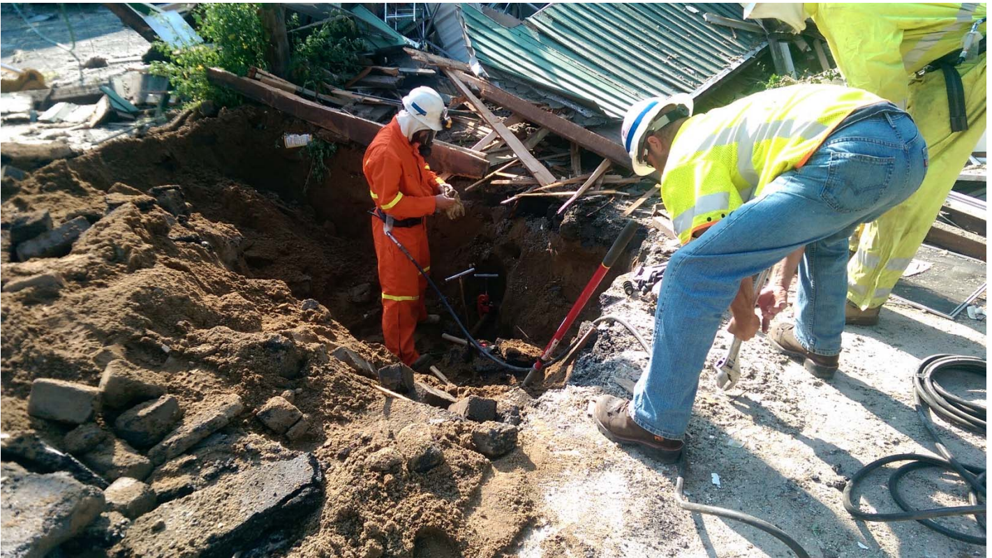
Photo 12 (8/10/14) – National Grid crews cutting the service at the main.
