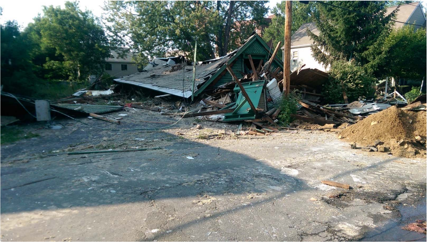
Photo 1 (8/10/2014) - 310 Paige Street after the explosion (Facing North).
