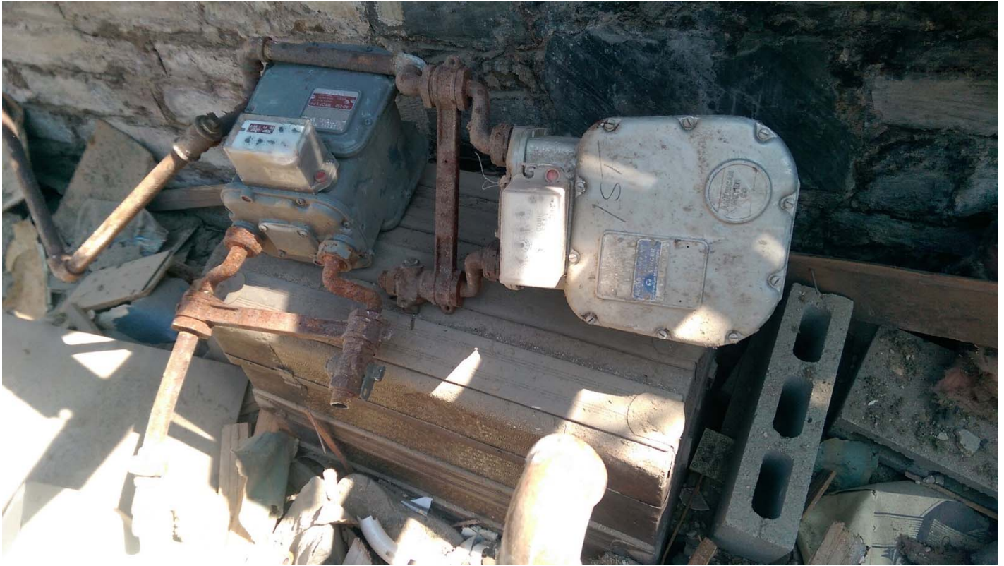
Photo 7 (8/11/2014) - Inside meters and service valves, after they were moved for observation.
