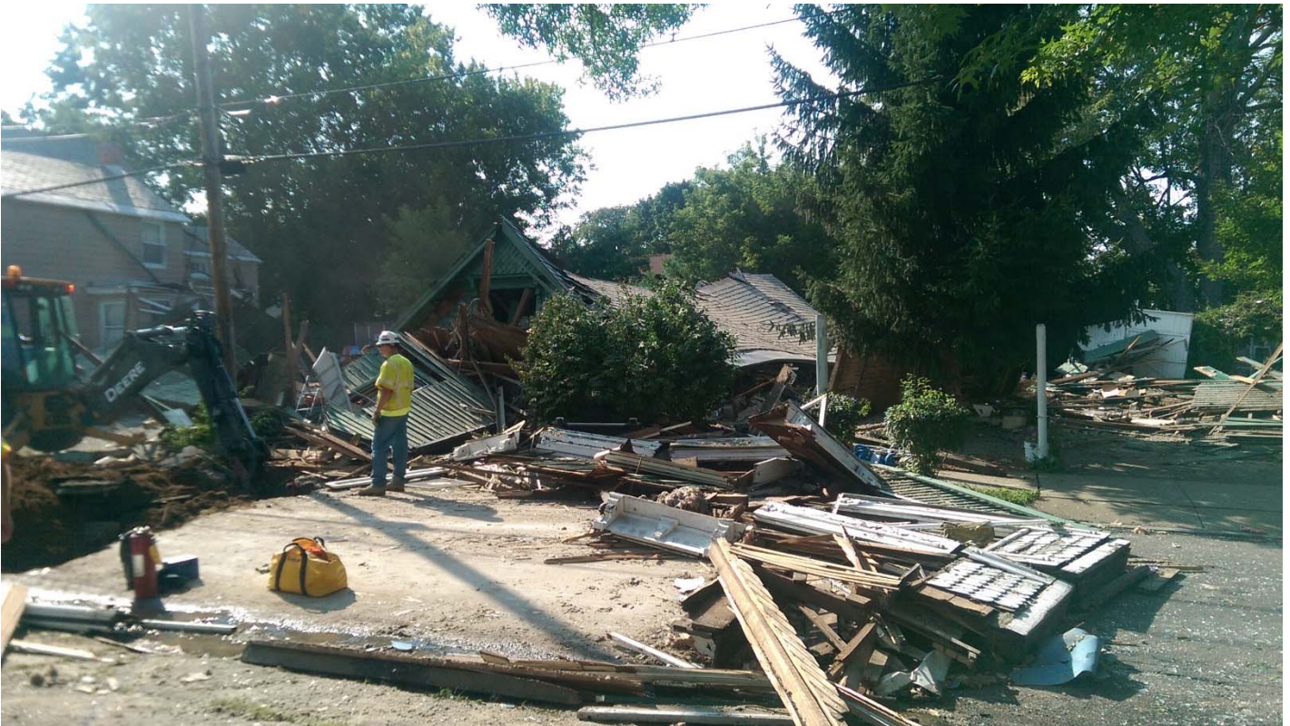
Photo 2 (8/10/2014) - 310 Paige Street after the explosion (Facing West).
