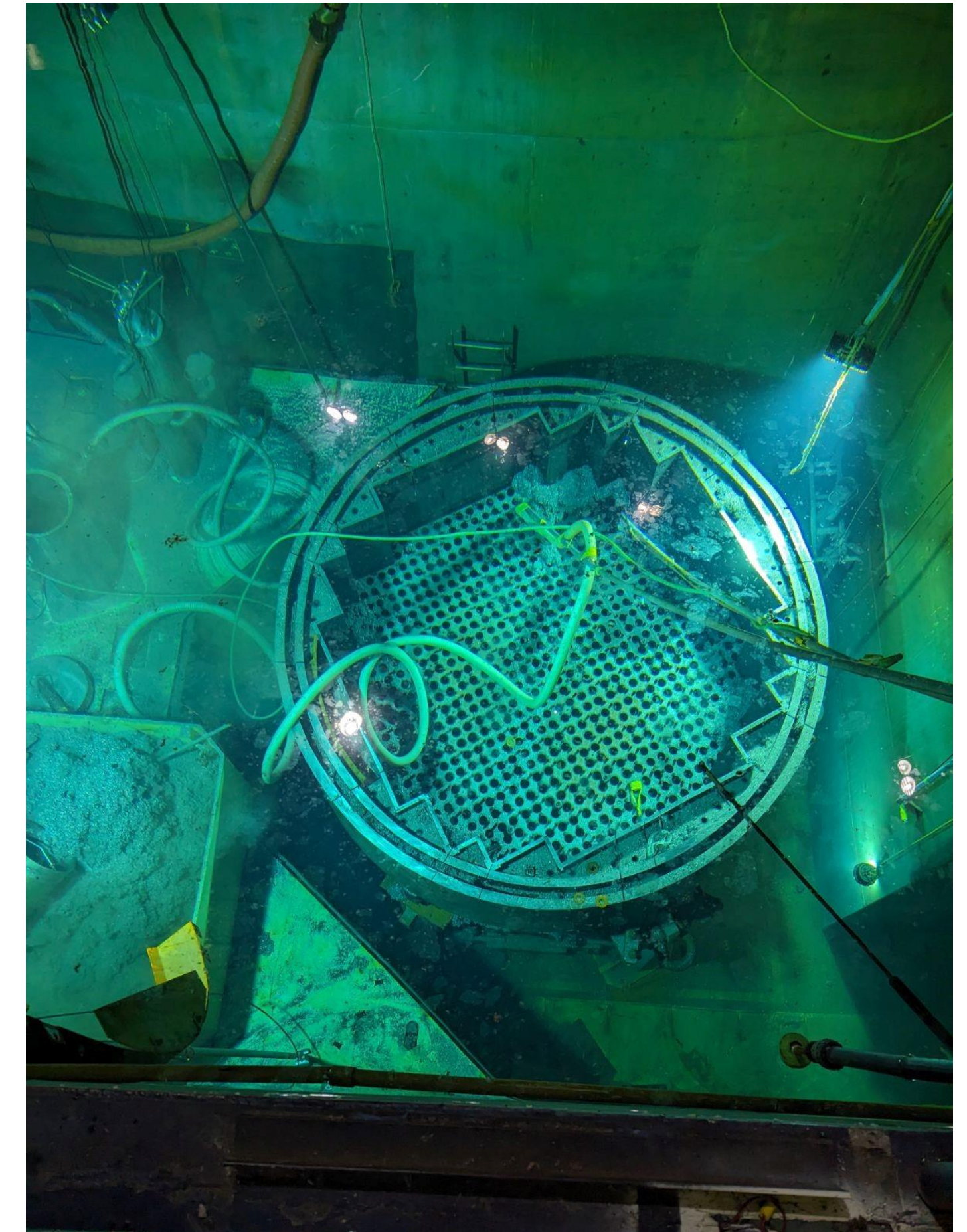
Unit 3 lower internals remaining for segmentation
