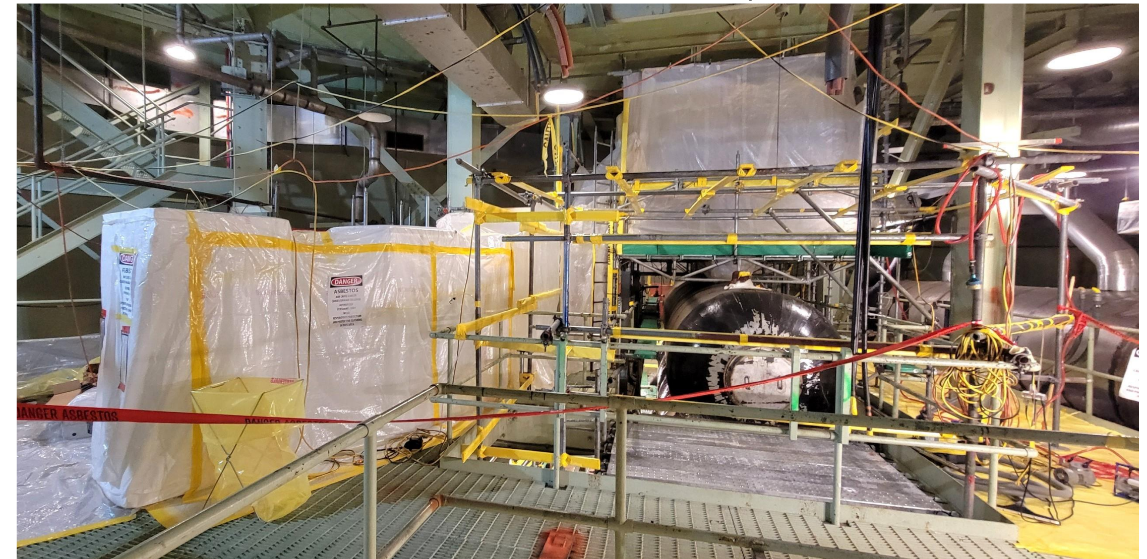
11 Boiler Abatement in Progress
