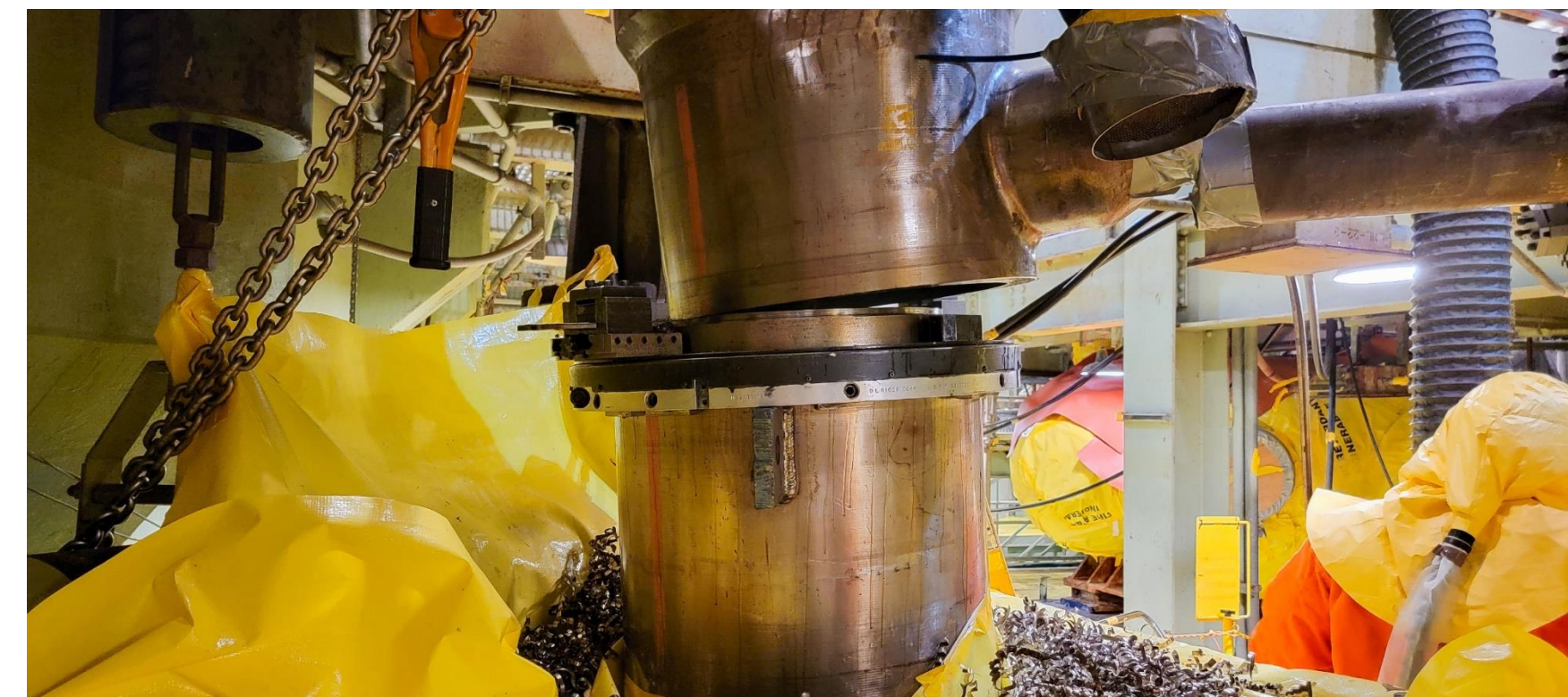
Example of RCS pipe cutting
