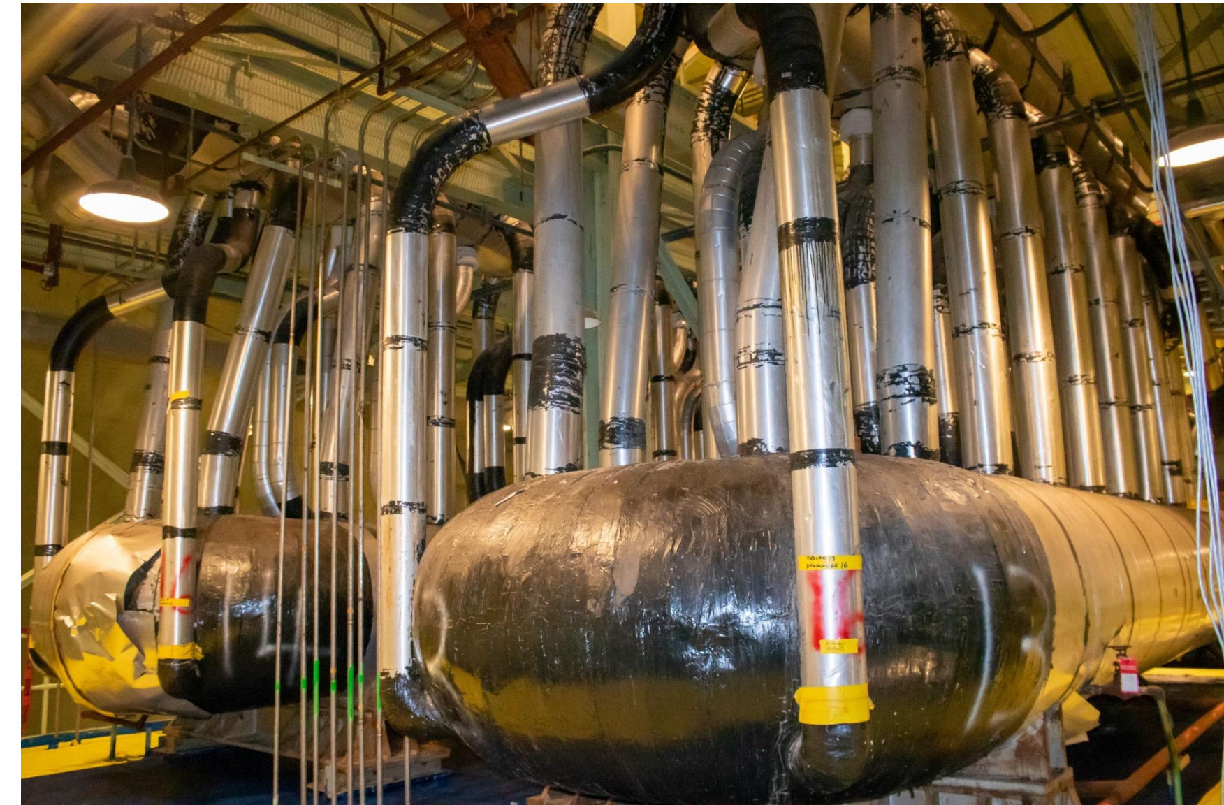
Unit 1 #13 & #14 Nuclear Boilers (Steam Generators)
