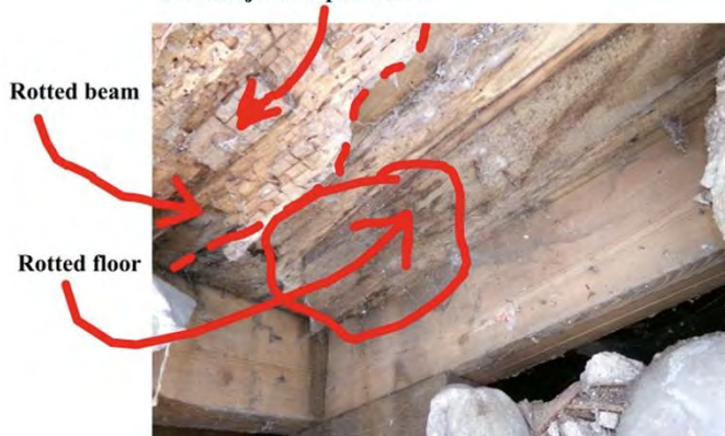
Mortise joint of post above
