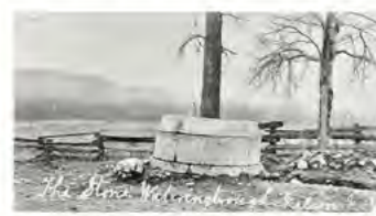
Another view of the Nelson Hill watering trough.
