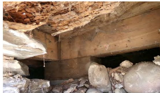
The 1970's (?) triple 2 x 10 beam about 3 feet in from the outer wall. The rotted old sill beam seen top left.
